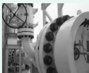
Replaced entire pig trap launcher barrel
