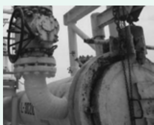
Damaged pig trap launcher barrel
