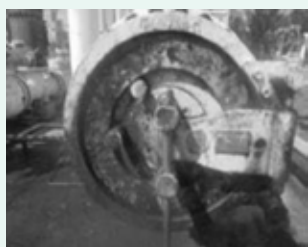
Corroded pig trap receiver door
